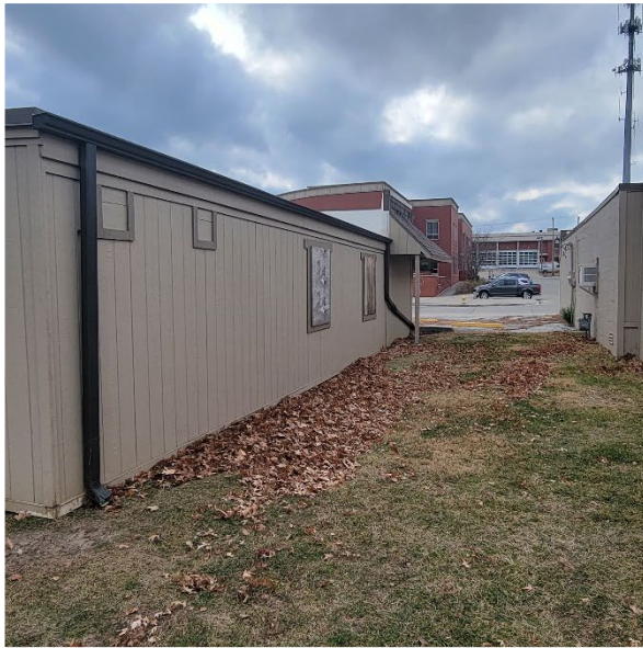
Interior to parcel 3 facing west
