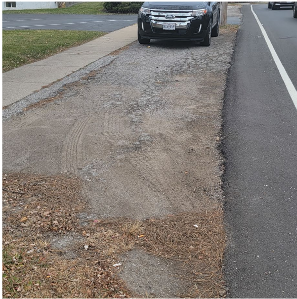
3rd Street facing east in front parcel 6
