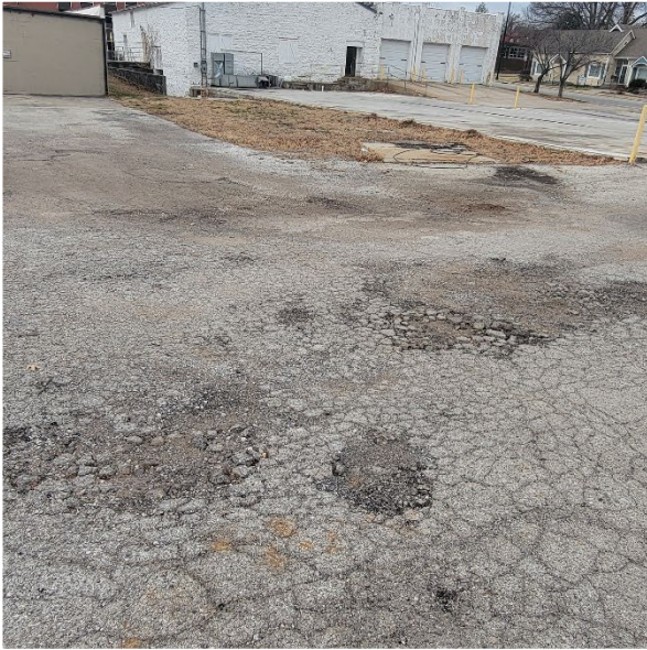
Interior to parcel 2 facing west
