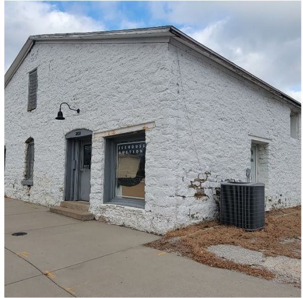
Green Street facing east in front of Parcel 3
