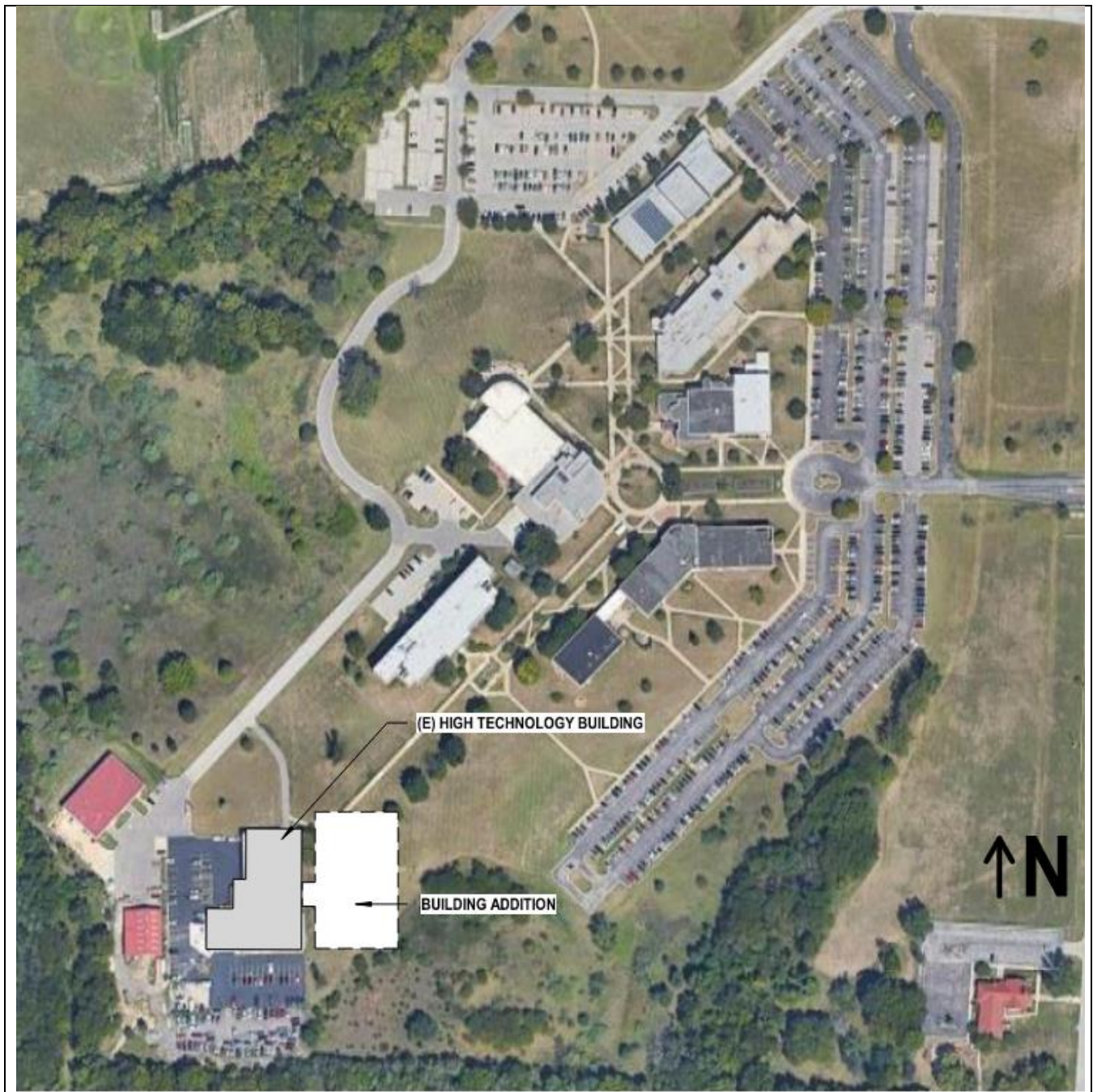
Figure 2 – Aerial of the MCC Longview Campus
