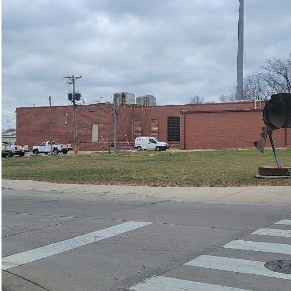
Southeast corner of 3rd and Green, Picture facing north
