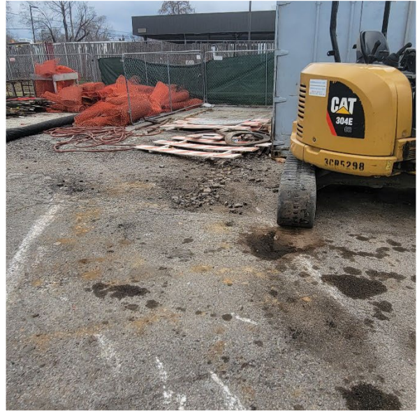
Interior to parcel 3 facing south
