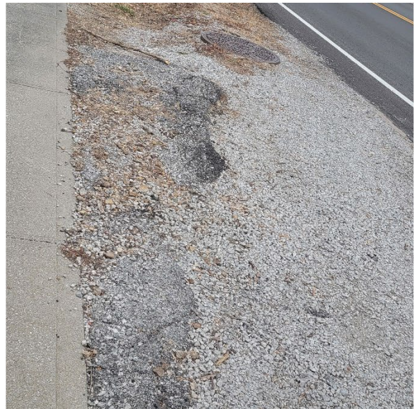
3rd Street in front of AT&T building
