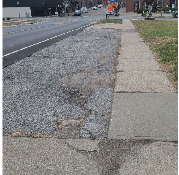
3rd Street in front of AT&T Building facing west
