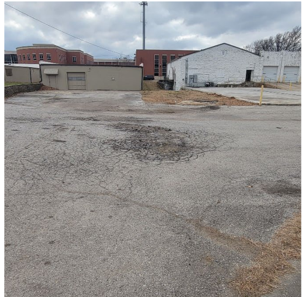
Johnson Street facing west in front of parcels 4 & 7
