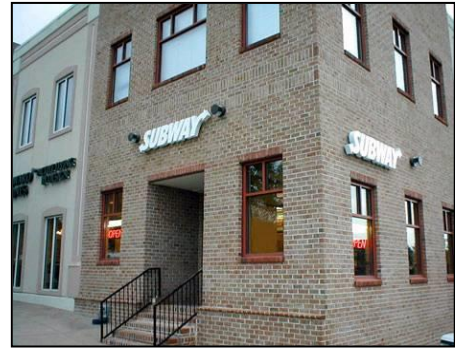
Fig. 6.480.B-28: Franchise design consistent with surrounding structures
