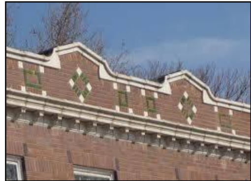
Fig. 6.480.B-5: Parapet wall screening roof mounted equipment
