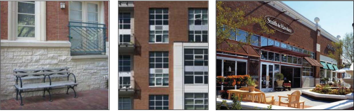
Fig. 6.480.B-29: Mix of building materials
