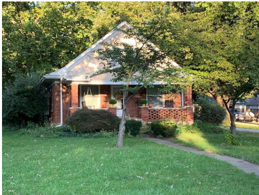
Existing Bungalow with Front Porch
