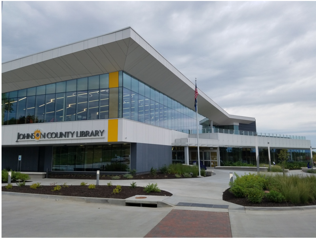
ACM panels on new Monticello Library, Overland Park, KS.
