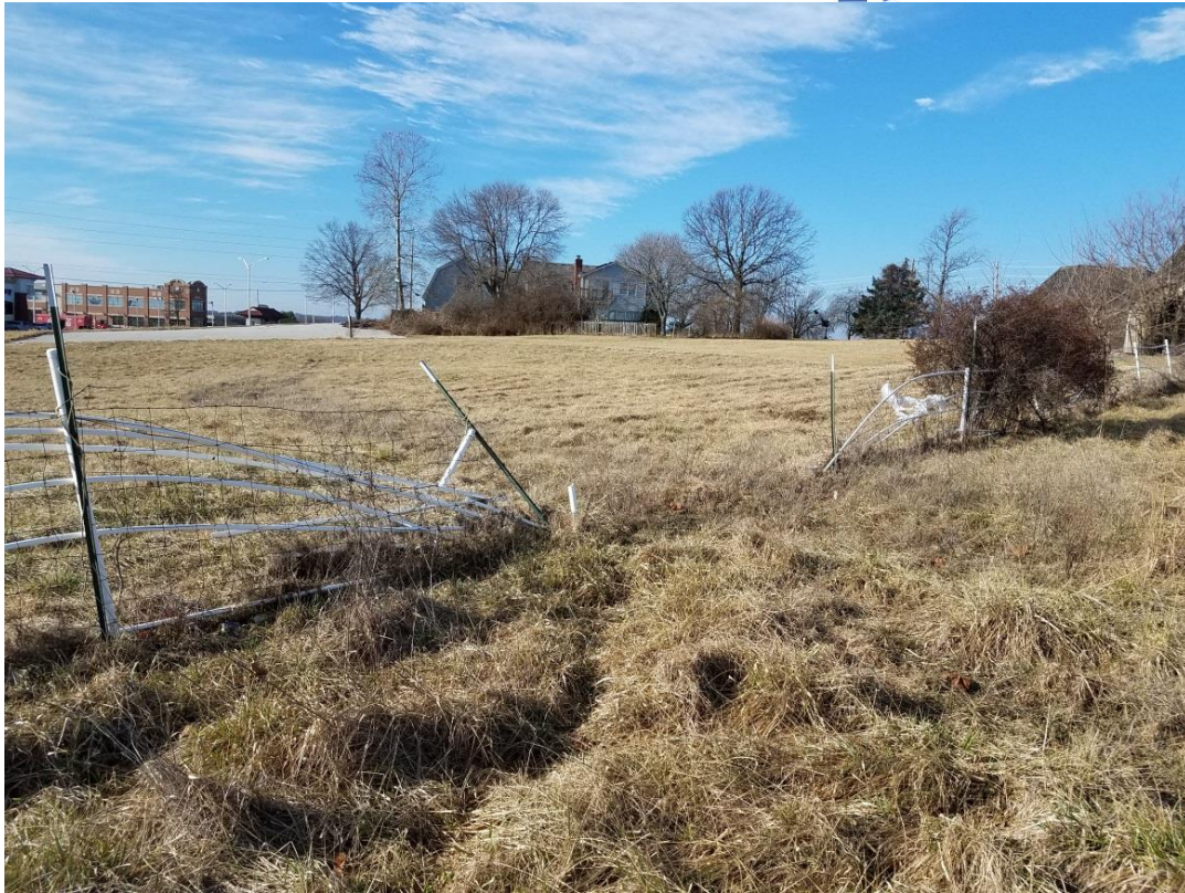
Photo 20 – Deteriorated/damaged fencing. Location - southern portion of the Redevelopment Area.
