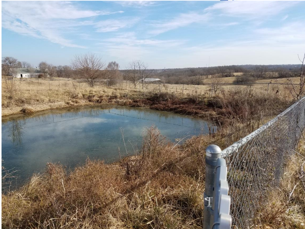
Photo 5 - Septic Pond located on Parcel 6. Note fencing surrounding pond, but open gate and easily accessible.
