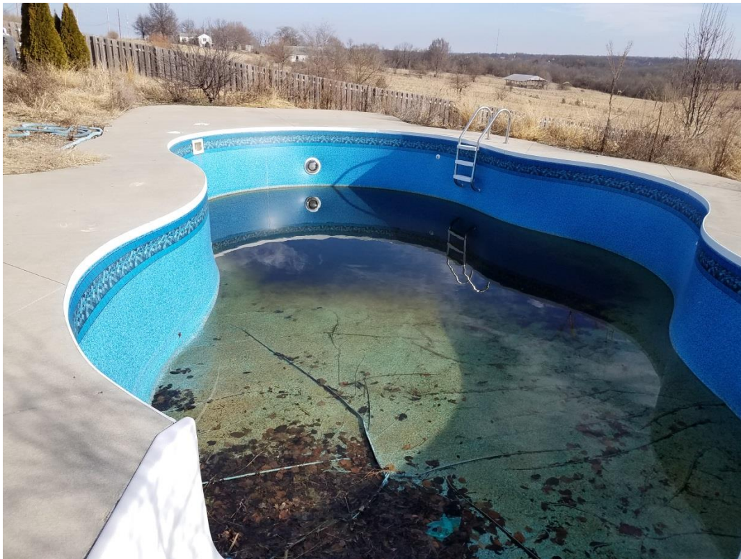
Photo 19 – View of partially filled pool (101 SW View High Drive. Note lack of safety equipment, signage.
