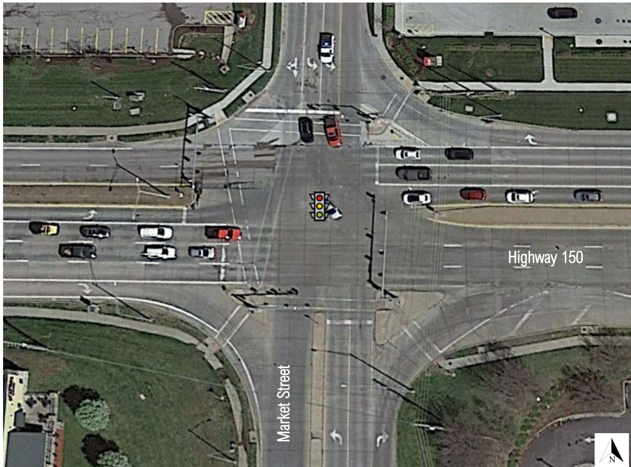
Figure 2: Aerial View of the Highway 150 and Market Street Intersection
