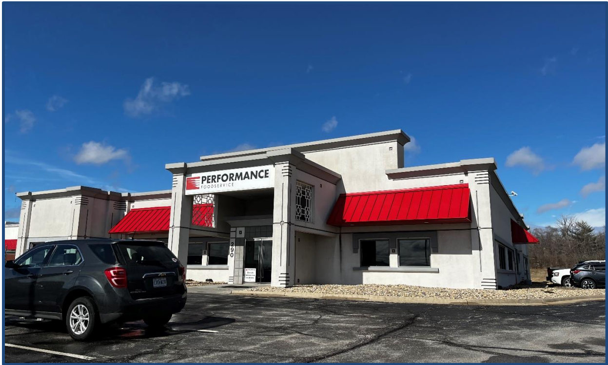
Representative exterior view of the existing property
