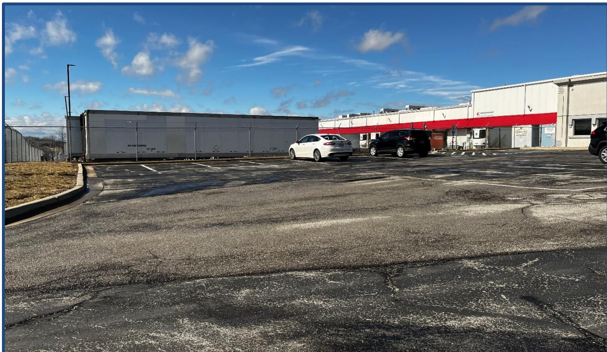
Representative site view of the existing facility
