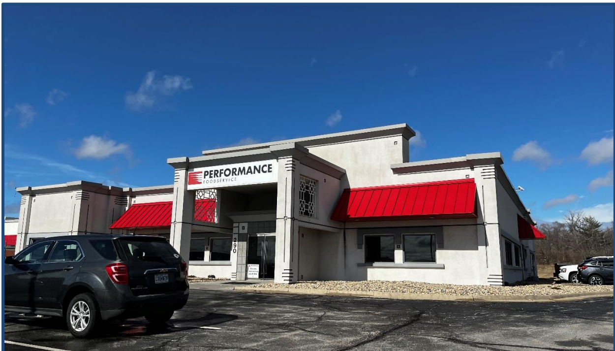
REPRESENTATIVE VIEW OF THE EXISTING FACILITY
