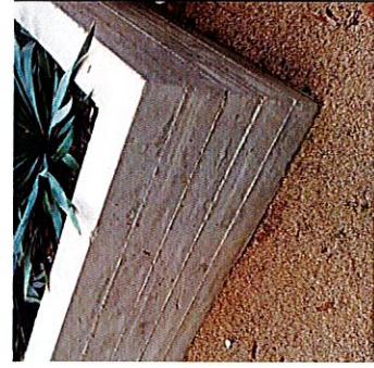
2 BOARD FORMED WALL IMAGE SCALE: 8/5
