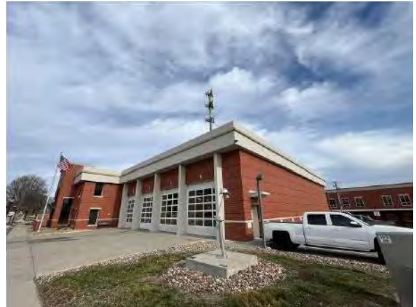
Photo #4 Facing N: Overview of site from S corner
