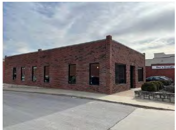
Photo #24 View of SE-adjacent vacant commercial building
