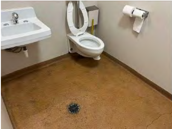
Photo #9 Typical on-site bathroom with floor drain
