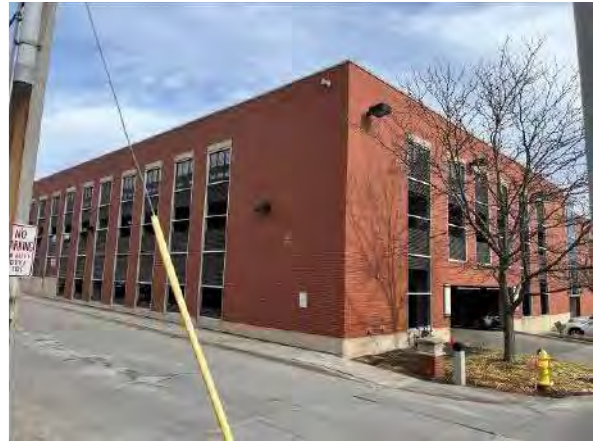
Photo #22 View of NE-adjacent parking garage
