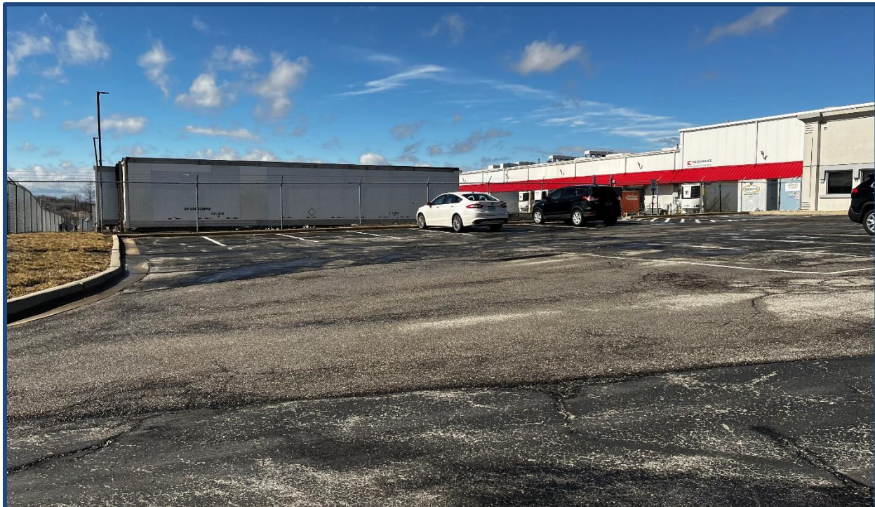
Representative site view of the existing facility
