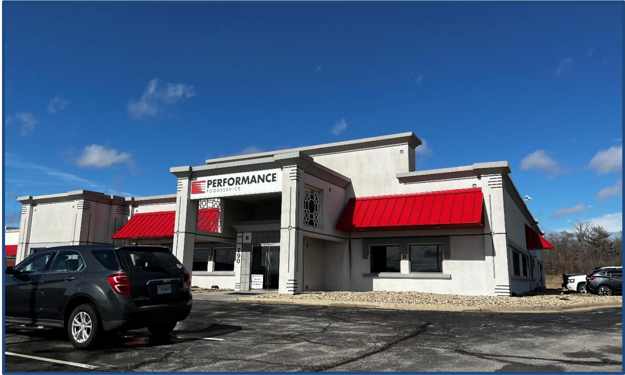
Representative exterior view of the existing property
