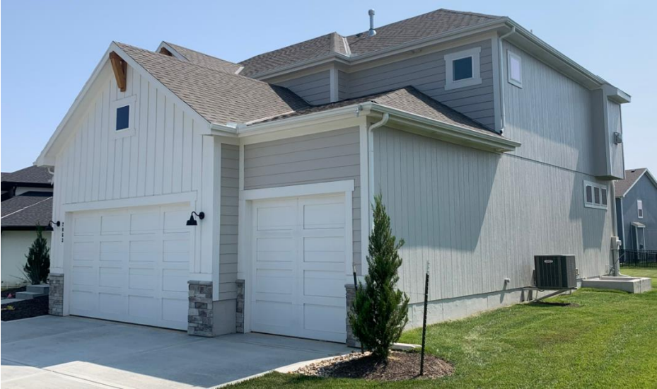
Figures 1 and 1 - Residence in Woodside Ridge with LP SmartSide board and batten and lap siding on front elevation and LP SmartSide panel on side elevation.
