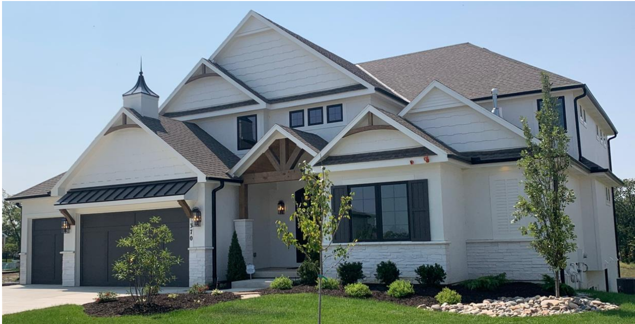
Figure 2 - Residence in Woodside Ridge with LP SmartSide shake siding on front elevation and LP SmartSide panel on side elevation.
