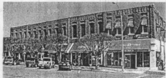
East Side of Main Street Between 2 nd and 3 rd Streets, 2003 Lee's Summit, Missouri Downtown History & Architecture Walking Tour
