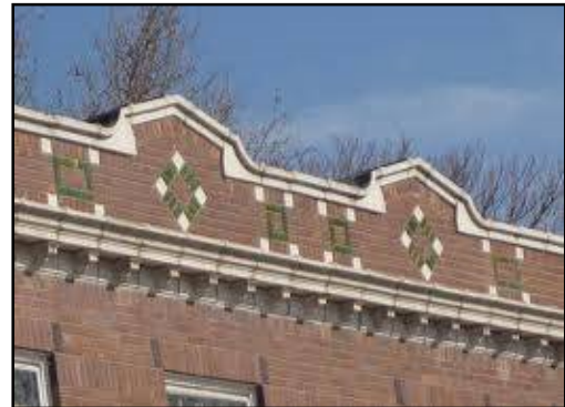
Parapet wall screening roof mounted equipment
