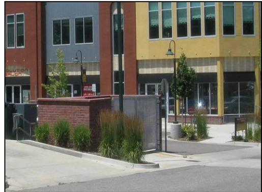
Refuse facility screening
