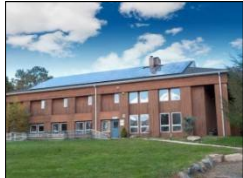
Commercial building with solar panels
