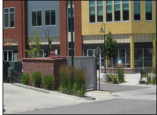
Refuse facility screening
