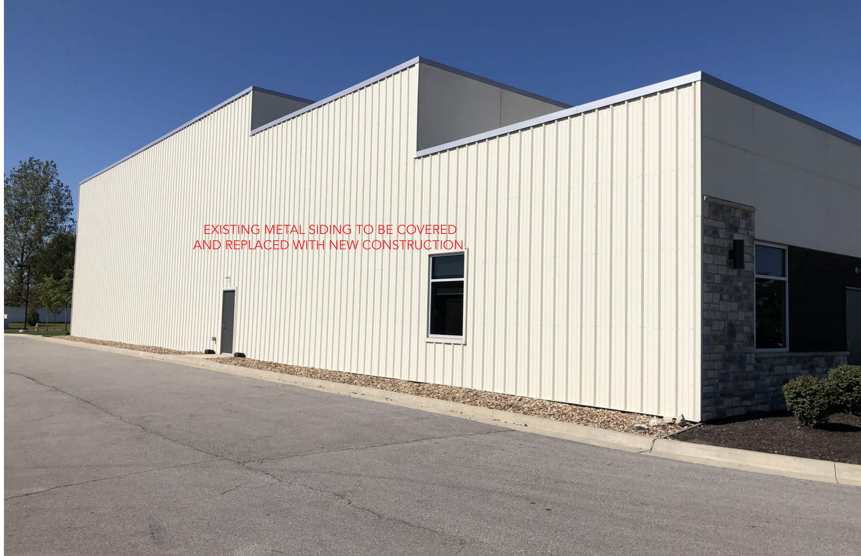
SOUTH ELEVATION (EXISTING)
