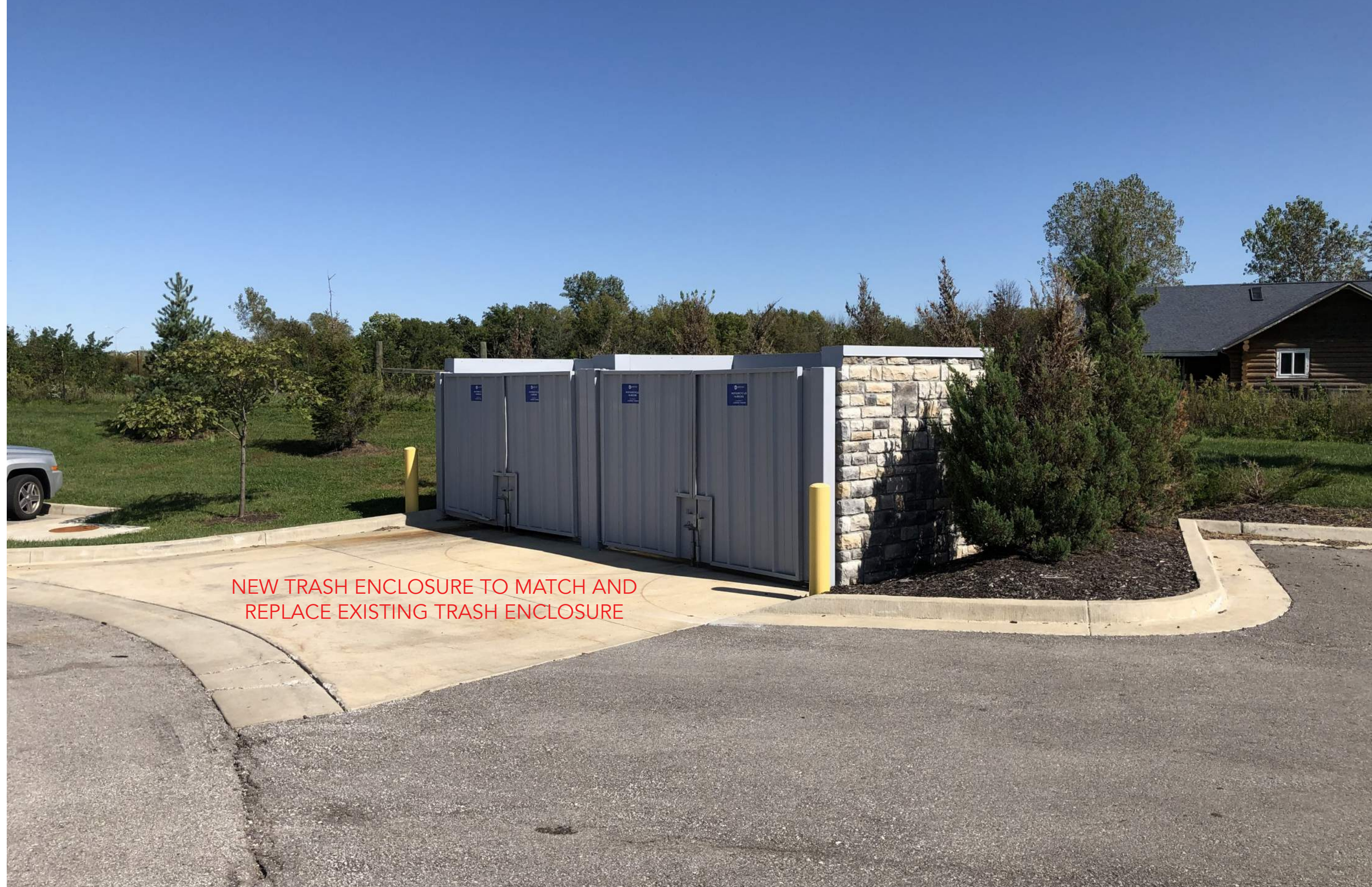
TRASH ENCLOSURE (EXISTING)
