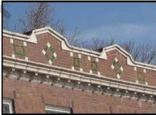
Parapet Wall Screening Roof Mounted Equipment
