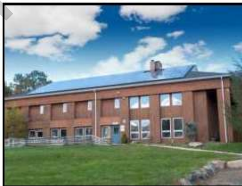
Commercial Building With Solar Panels
