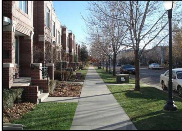
Figure 5.510.B-11: Ground-Floor Unit Entrances
