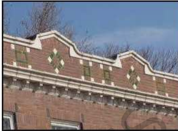
Figure 5.510.B-5: Parapet Wall Screening Roof Mounted Equipment
