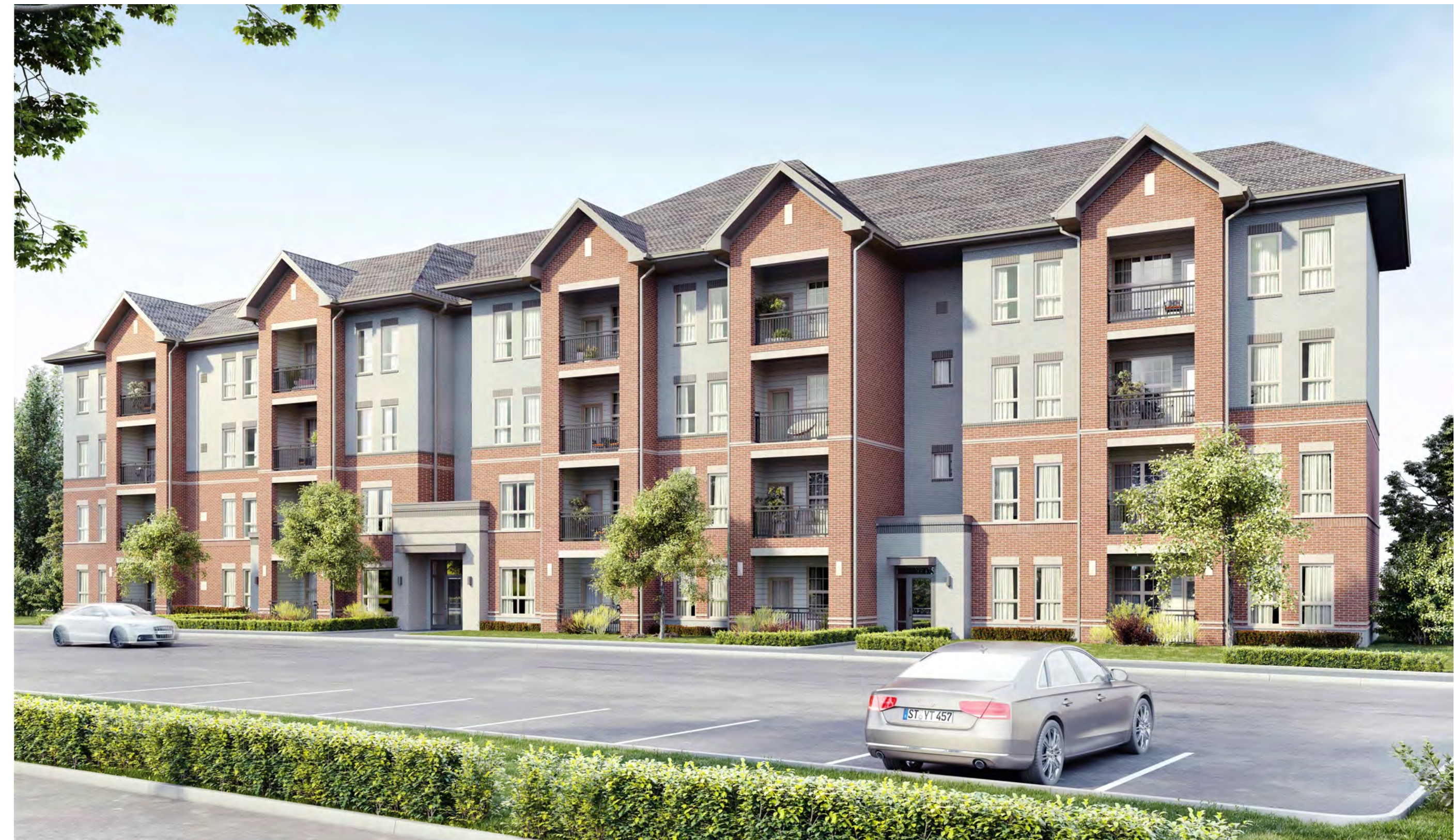
RESIDENTIAL BUILDING (FRONT)
