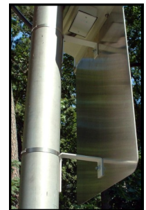
Installed regulatory speed limit sign using extender bracket set
