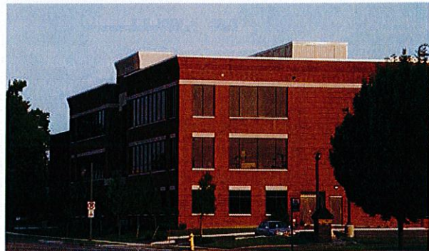
The Ohio State University Foundation - Columbus, Ohio
