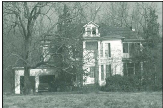
Fig. 6.480.B-9: Historic structures in the M-150 Corridor feature clean lines and simple design details.
