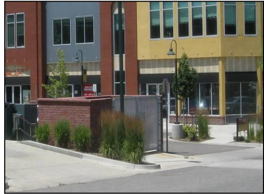
Fig. 6.480.B-7: Refuse facility screening
