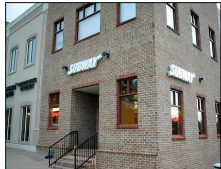
Fig. 6.480.B-28: Franchise design consistent with surrounding structures
