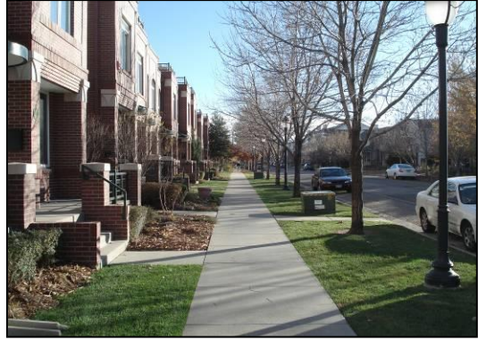
Fig.6.480.B-15: Ground-floor unit entrances
