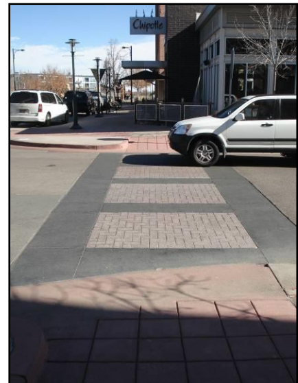
Fig. 6.480.B-3: Decorative materials for pedestrian crossings
