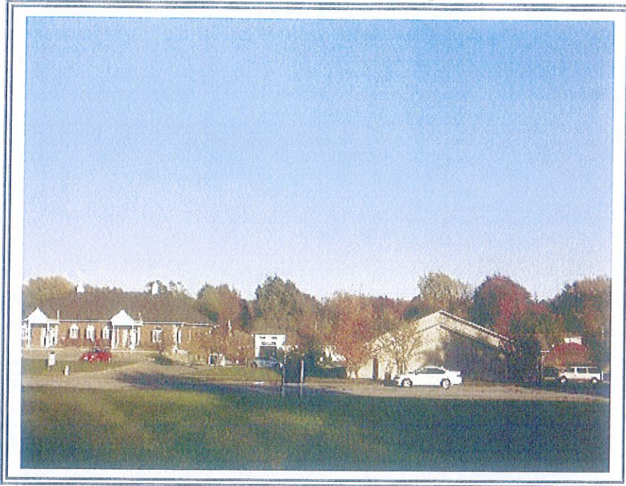
Site Facing East
