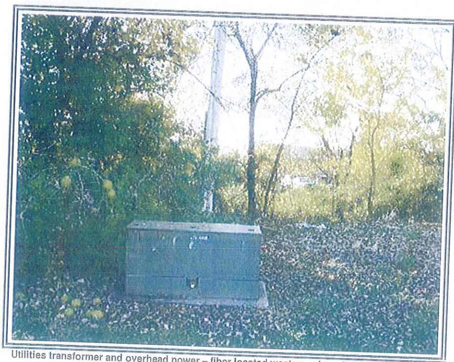
Ingress / Egress off of NW Executive Pkwy South side of parcel
