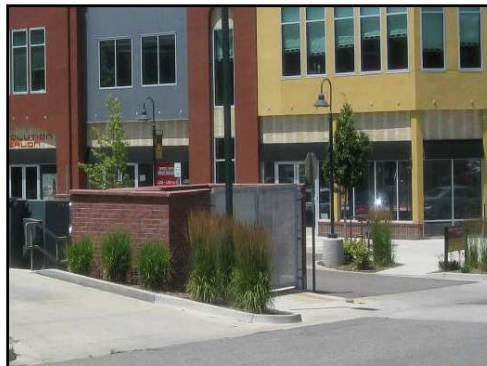
Refuse Facility Screening
