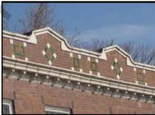
Parapet Wall Screening Roof Mounted Equipment
