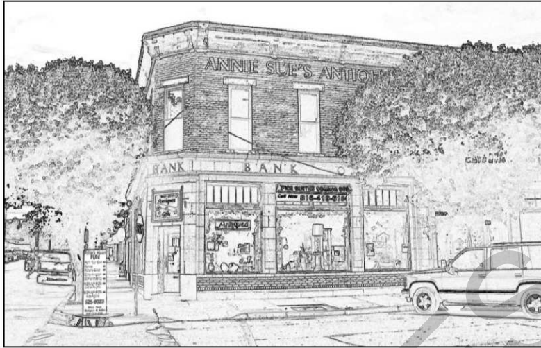
Two-story Tapestry Brick commercial building at 228 SW Main Street. This building's storefront was remodeled in the early 20th century with terra cotta and large display windows. At the roofline is a sheet metal cornice.
