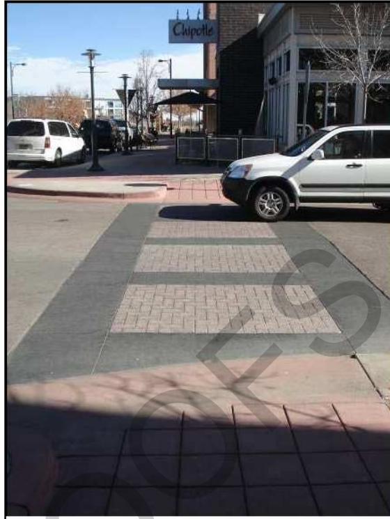
Figure 5.510.B-3: Decorative Materials for Pedestrian Crossings
