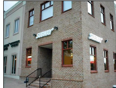
Fig. 6.480.B-28: Franchise design consistent with surrounding structures
