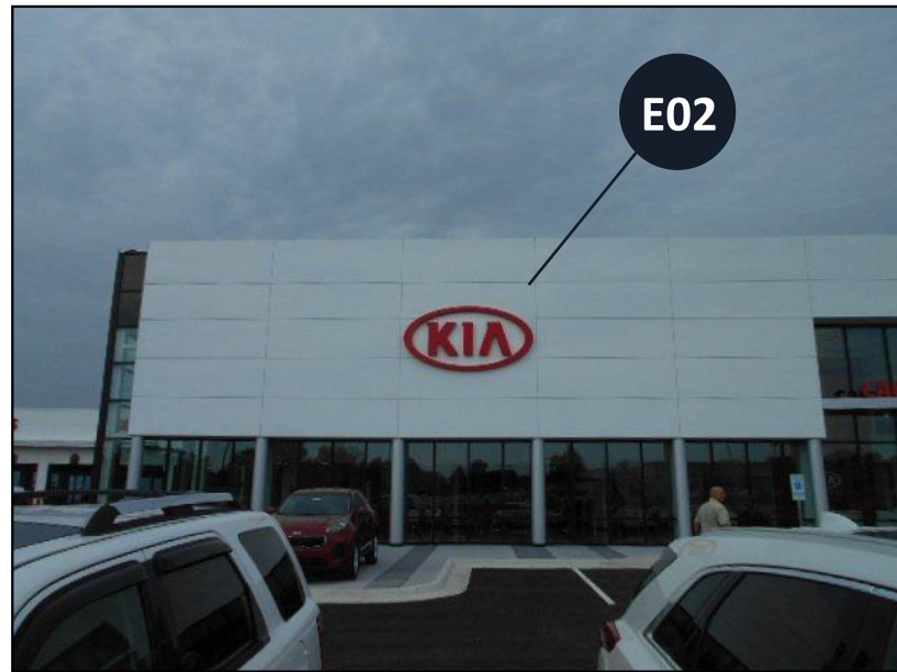
NOTE: PSG to remove & scrap existing signs.
