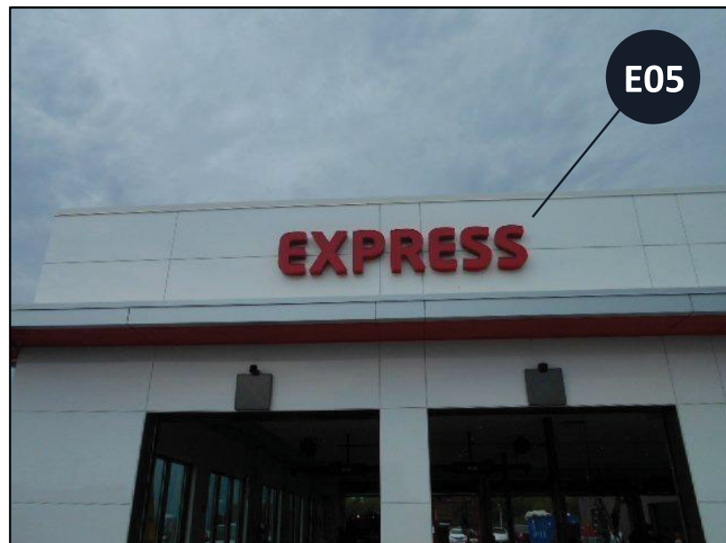
NOTE: PSG to remove & scrap existing signs.
