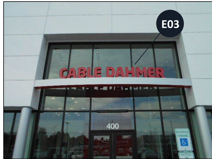
NOTE: PSG to remove & scrap existing signs.
