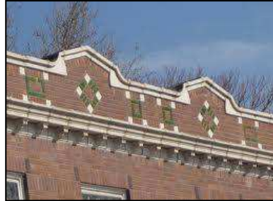
Fig. 6.480.B-5: Parapet wall screening roof mounted equipment
