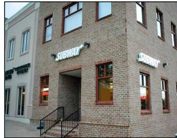
Fig. 6.480.B-28: Franchise design consistent with surrounding structures
