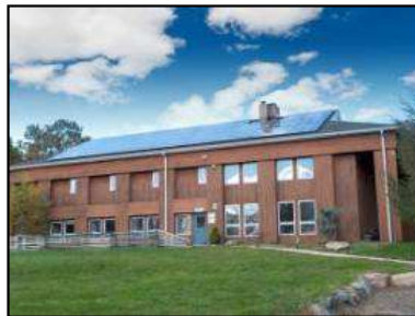
Fig.6.480.B-34: Commercial building with solar panels
