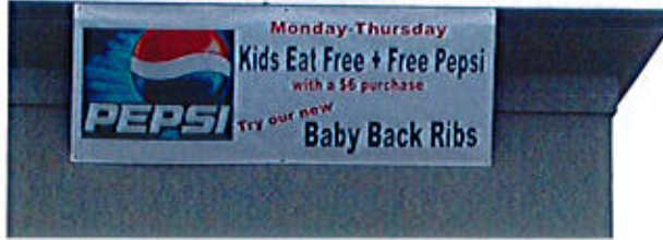
Banner attached to structure
